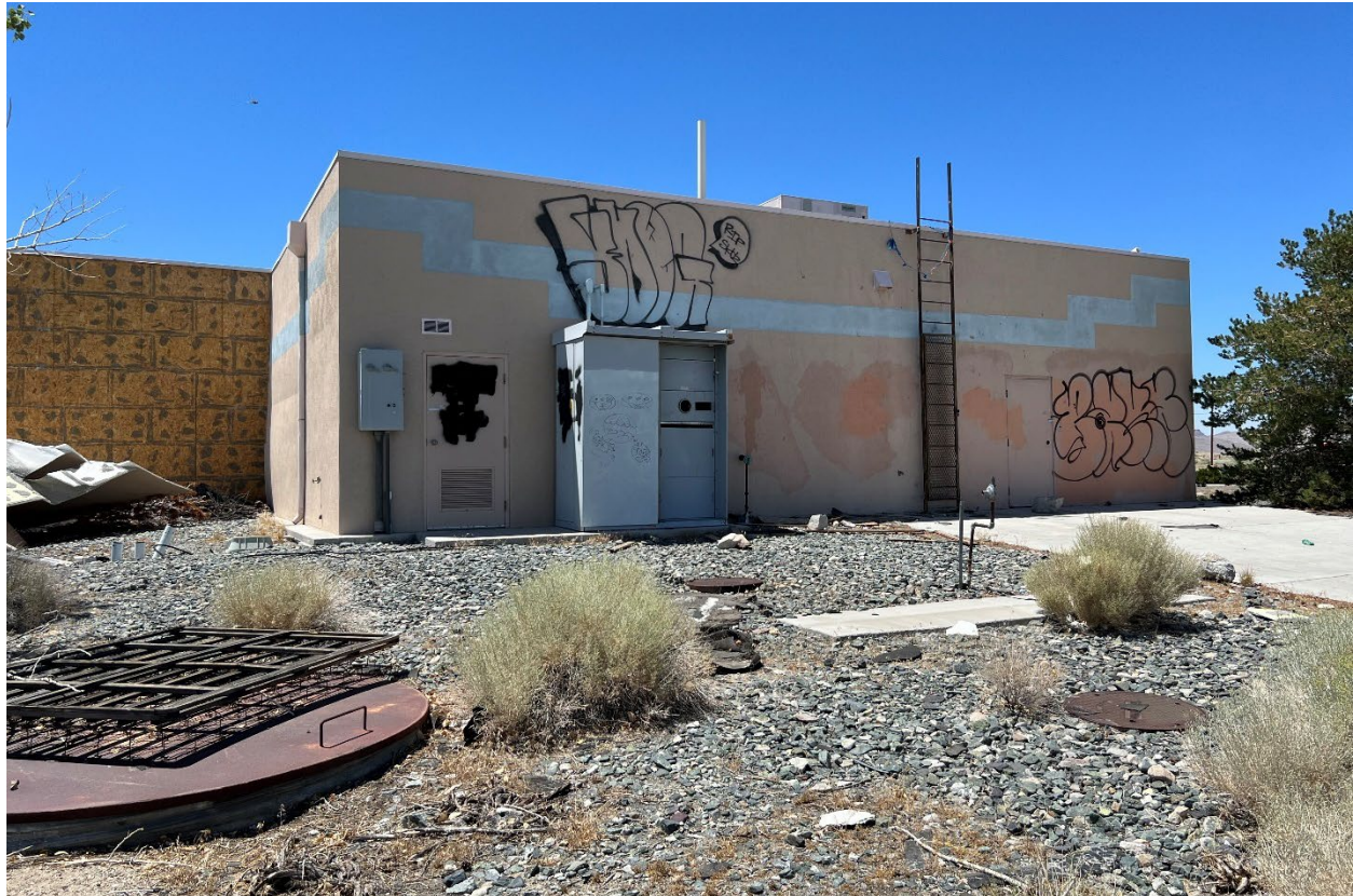
Figure 9. Rear (east) side of the building showing electrical boxes and roof access.
