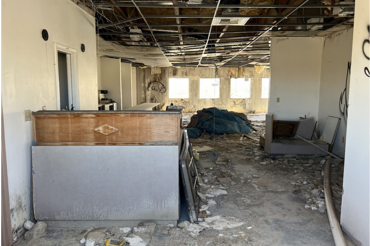
Figure 11. Opposite angle looking south at the interior common area from Figure 6
